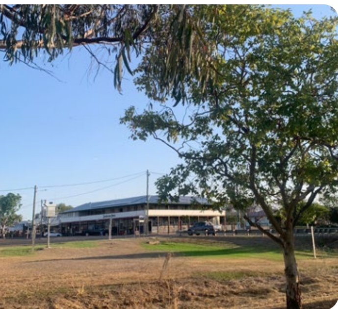
Corner of Dalby and High st (above + above right): Visual connection to main street from Lions Park, across the road from Jandowae Motel and Athlone Cottage.
